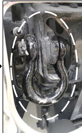
Figure 2c: Before removing tow shackles
